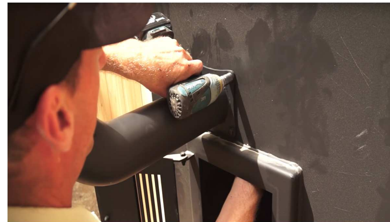
WB-4. Using a wrench to hold the nut on the inside, tighten the bolts completely with the drill or a wrench.
