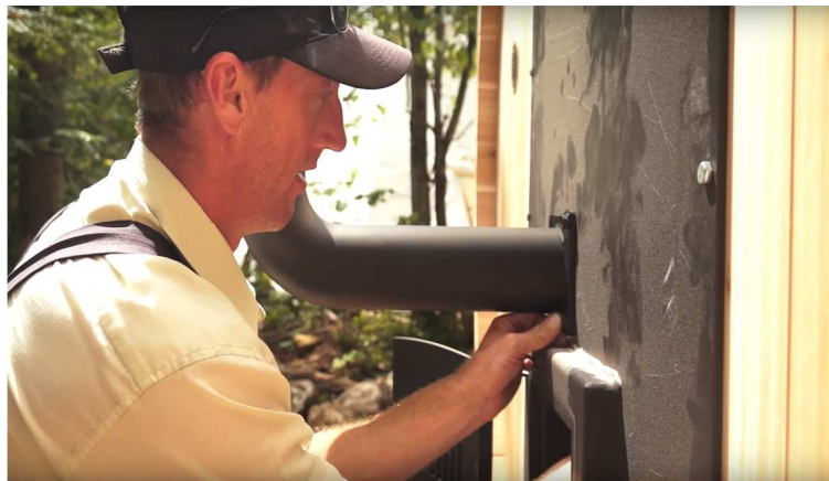
WB-3. Attach chimney elbow to the wood burning stove by pushing provided bolts into place and securing with nuts on the other side.
