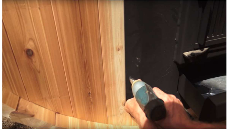
WB-2. Secure with provided lag screws. * Do not overtighten as this will strip the screws.
